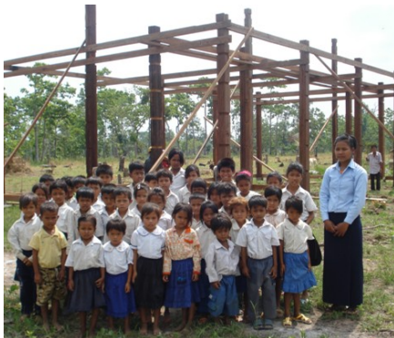
STUDENTS IN FRONT OF THE NEW SCHOOL DURING CONSTRUCTION.
